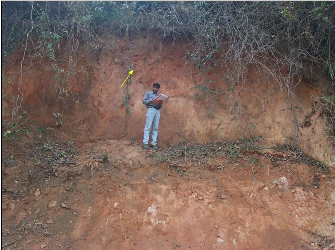
Photo 56: View of the debris slide on the
