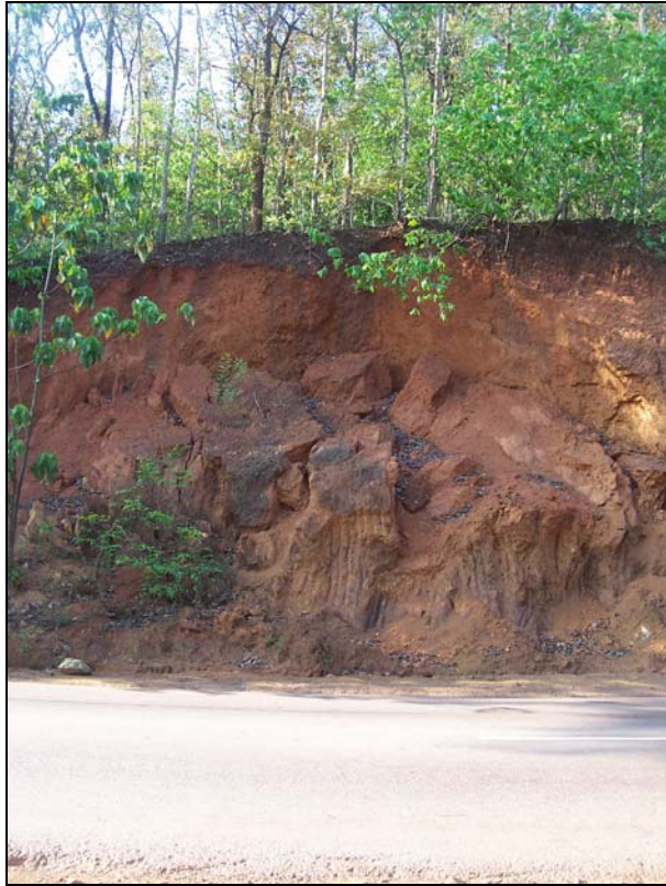
Photo 110: The side view of the debris slide showing steep slope angle.
