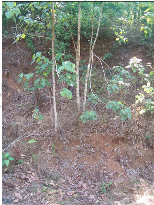
Photo 77: The view of the unstable crown portion of debris slide
