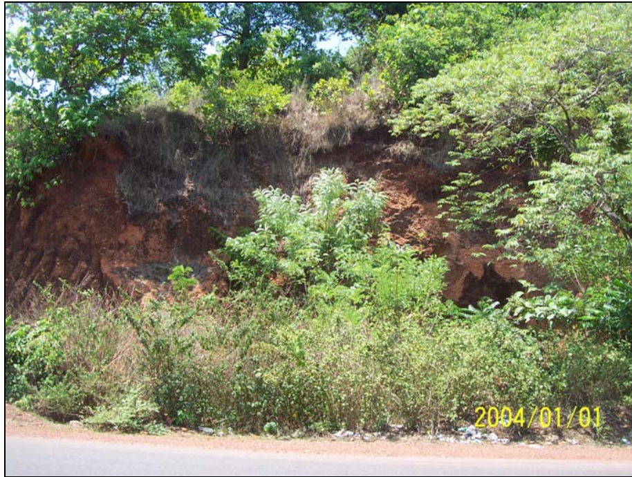
Photo 127: The side view of the reactivated, debris slide with unstable crown
