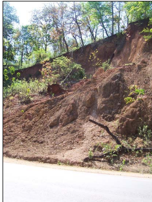
Photo 96: The view of the debris slide with unstable crown
