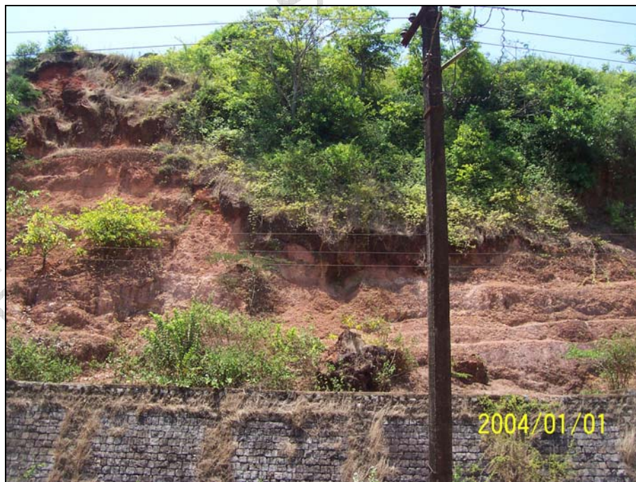
Photo 124: The plan view of the reactivated, debris slide with no protection at the mid slope and is likely to slide again
