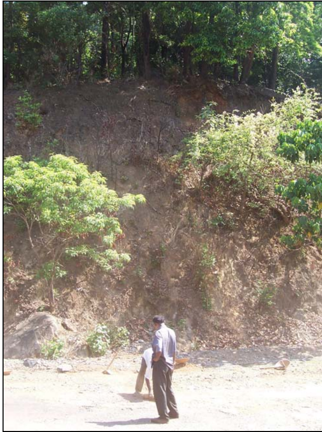
Photo 68: The plan view of the debris slide with exposed bed rock
