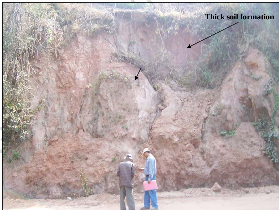
Photo 12: The circular failure of the slide with the exposed bedrock (weathered granite)
