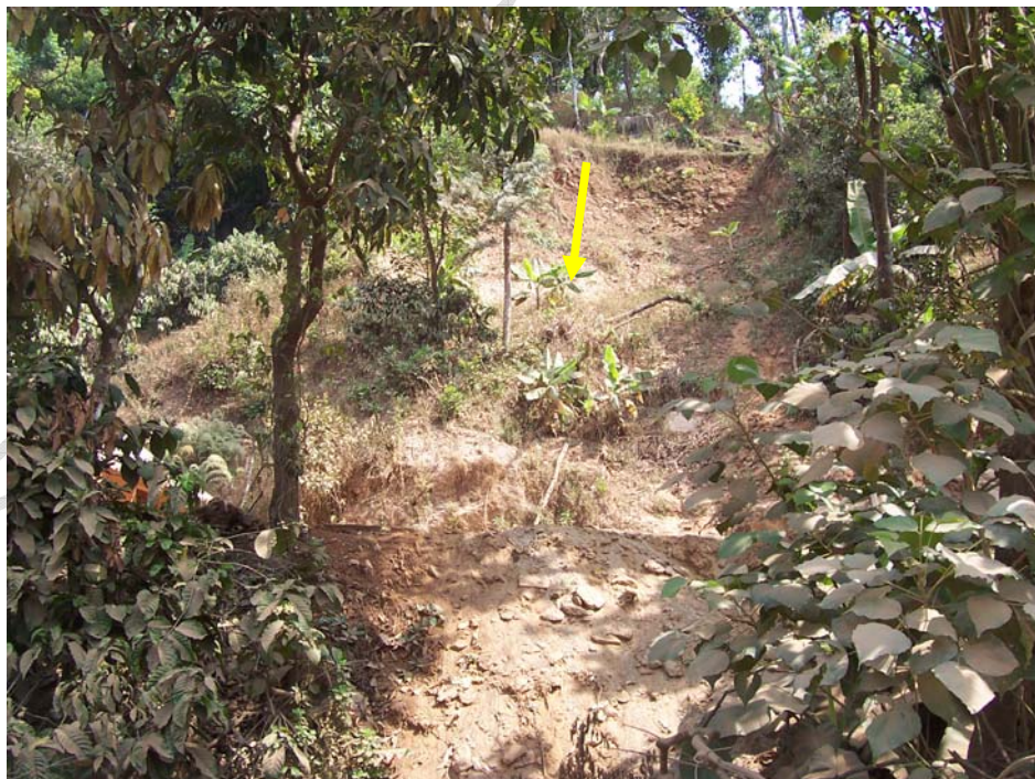
Photo 54: Plan view of the reactivated debris slide which has crown height of 2m.
