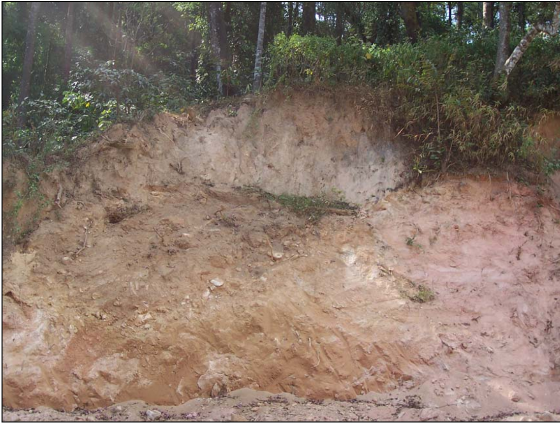
Photo 55: Plan view of the debris slide which has crown height of 2m and crown width of around 8 m.
