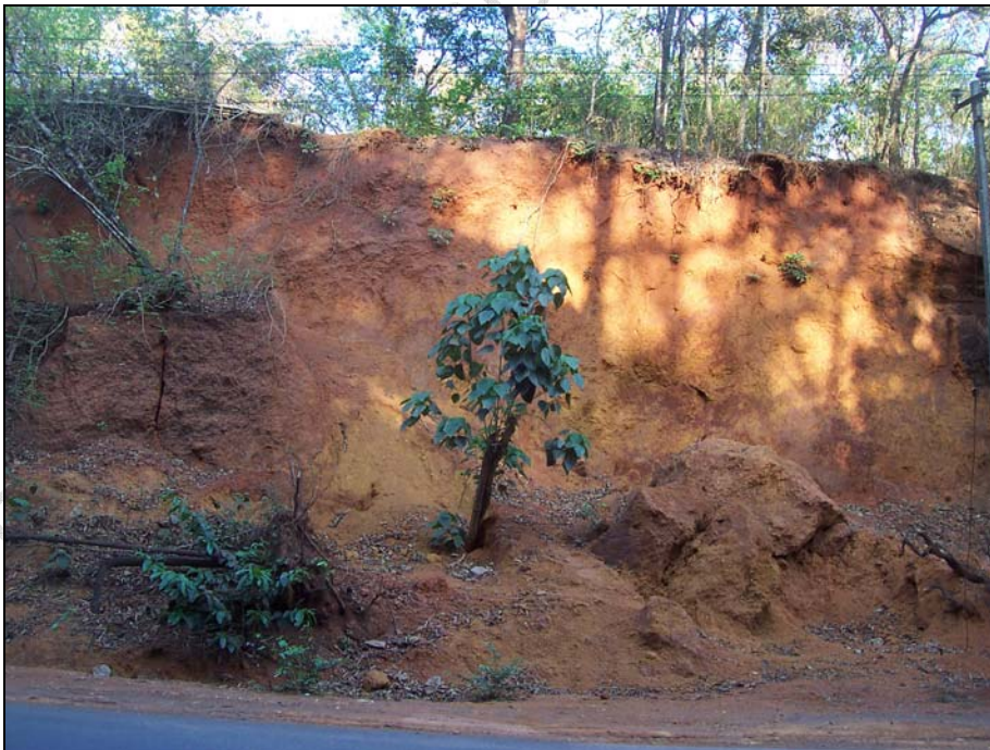
Photo 107: The side view of the debris slide showing steep slope angle.
