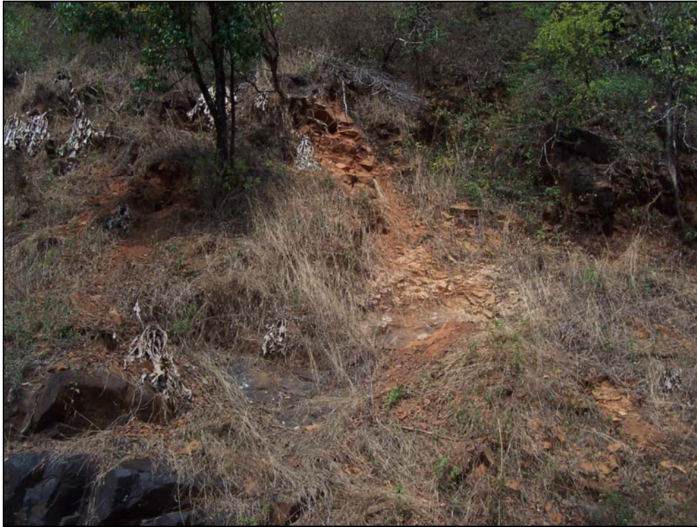
Photo 84: The plan view of the rock slide with loose boulders accumulated at the toe of the slide.
