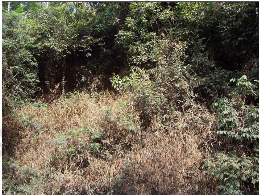
Photo 52: View of the debris slump which is covered by small trees
