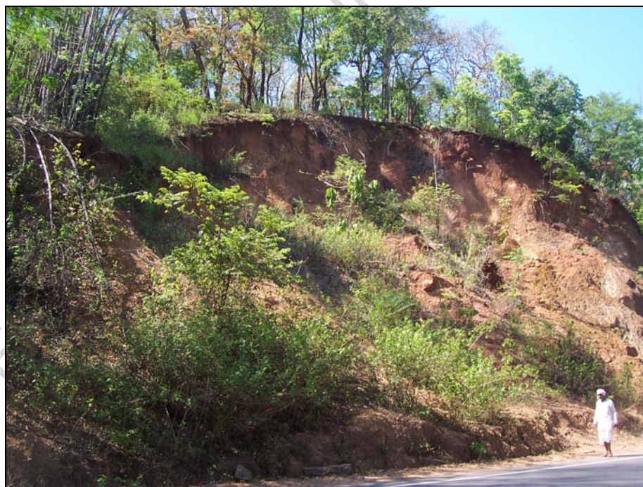
Photo 97: The side view of the debris slide
