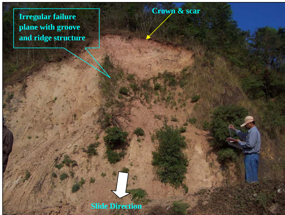
Photo-1: The plan view of the landslide along Madikere-Mangalore road section (SH88)
