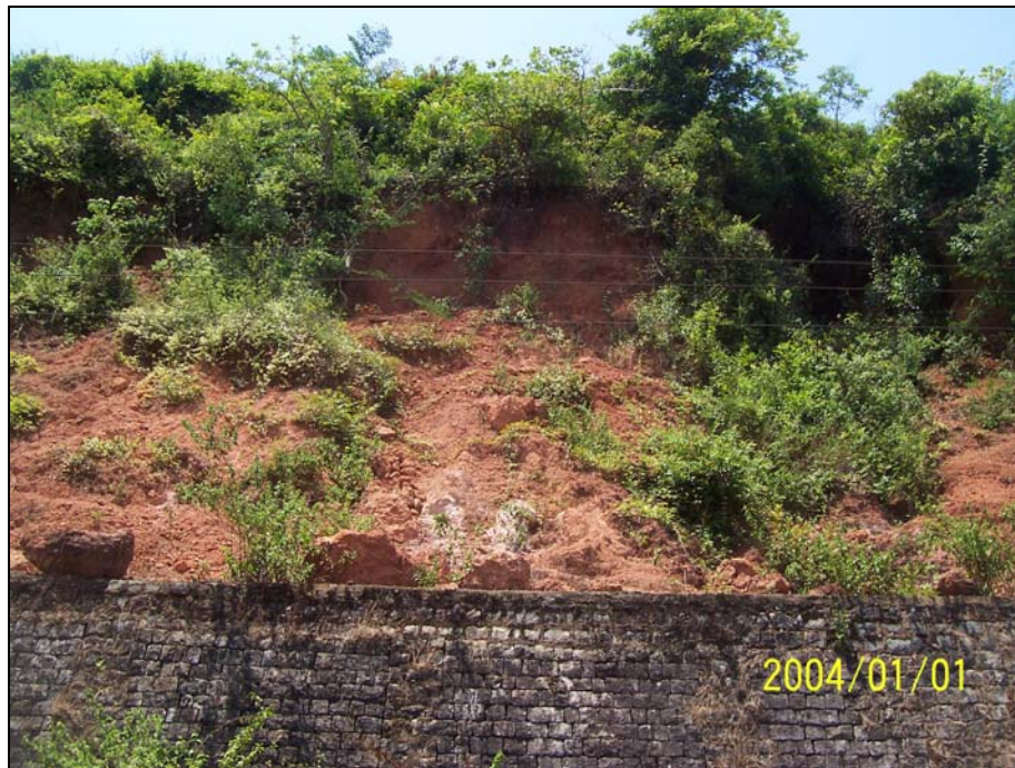
Photo 123: The plan view of the reactivated, debris slide with unstable crown. No protection at the crown
