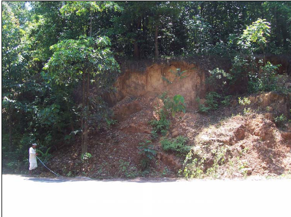
Photo-86: The plan view of the debris slide with unstable crown.
