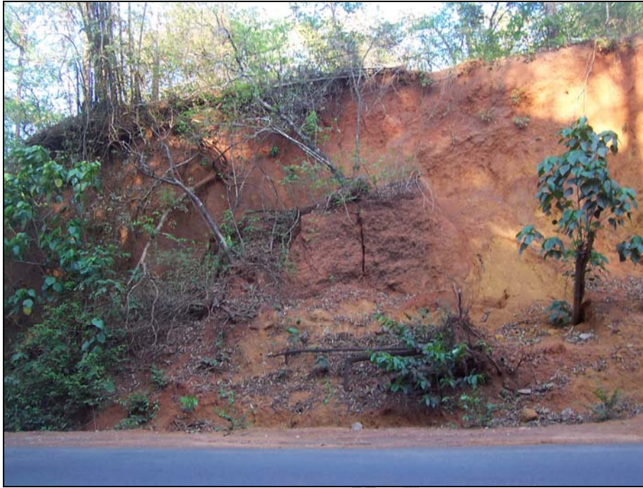
Photo 106: The side view of the debris slide showing steep slope angle.
