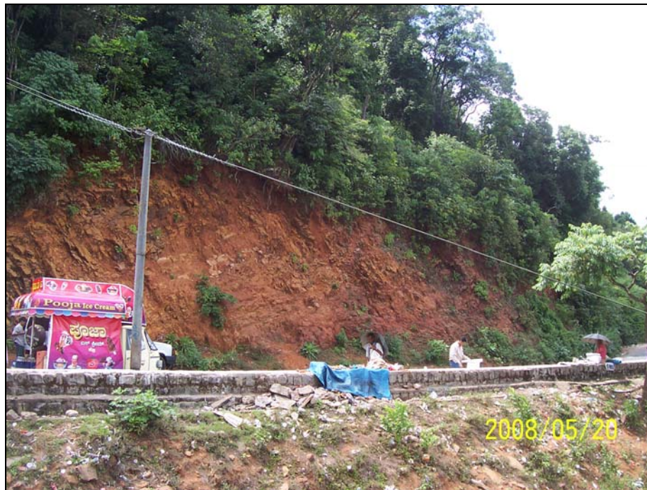
Photo 115: The side view of the debris slump
