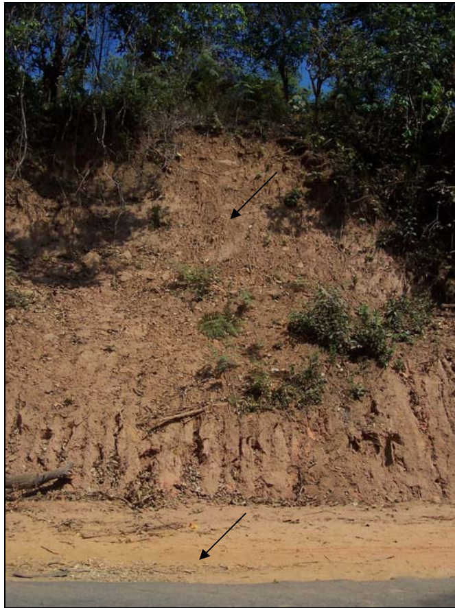
Photo 21: View of the slide plane and the accumulation zone
