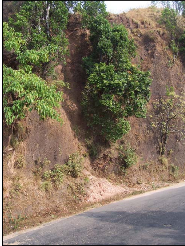
Photo 47: View of the rock slide with trees on the crown and slide plane
