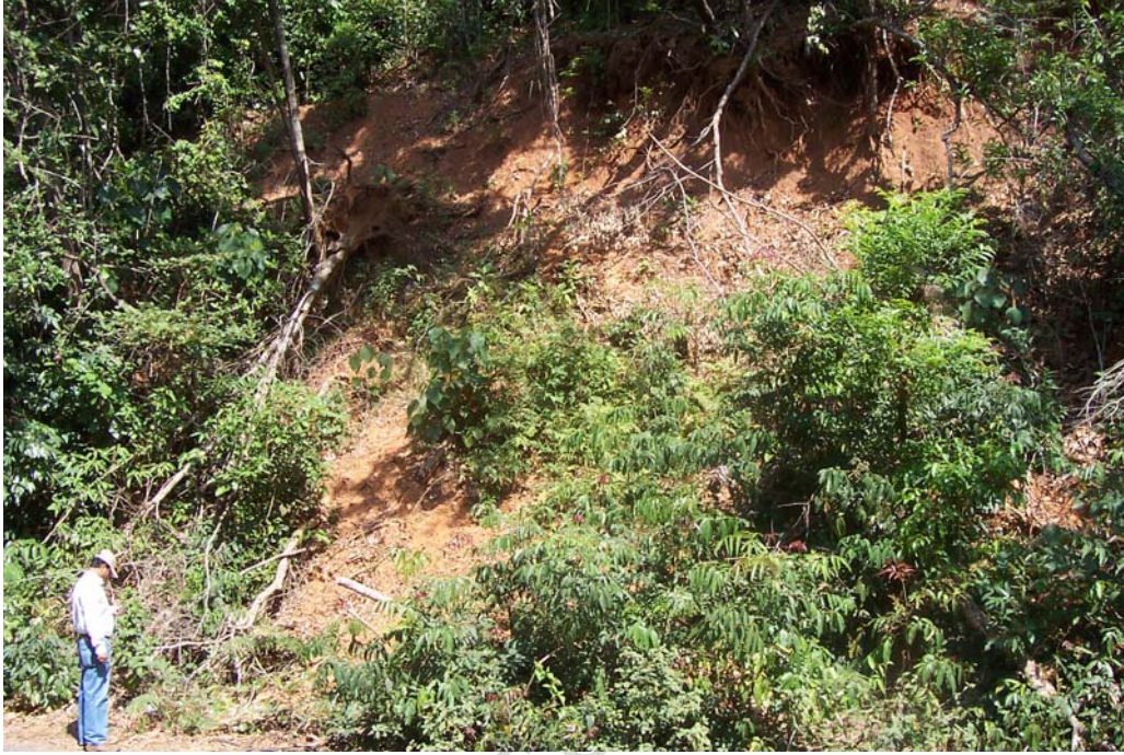
Photo-112: View of the debris slide with slided material
