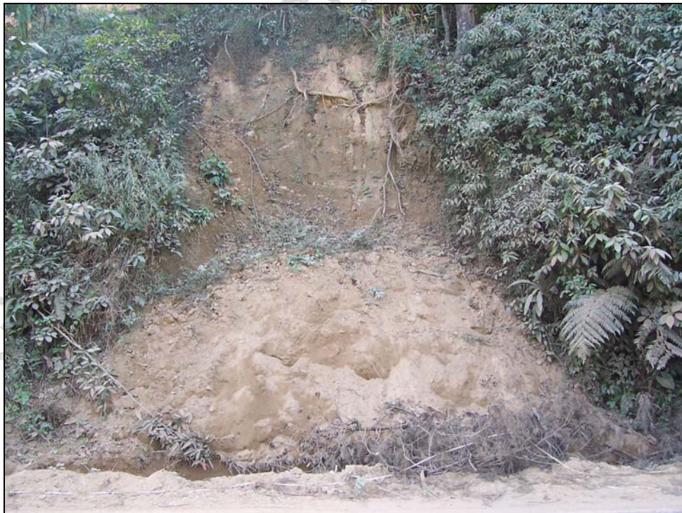
Photo 39: The plan view of the debris slide with zone of accumulation
