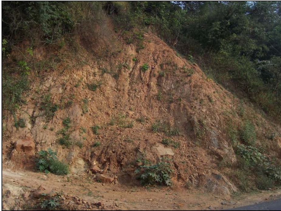
Photo 43: Plan view of the reactivated slide with exposed weathered granite
