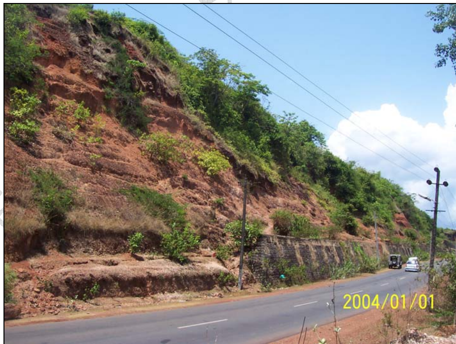
Photo 126: The side view of the reactivated, debris slide with steep slope angle
