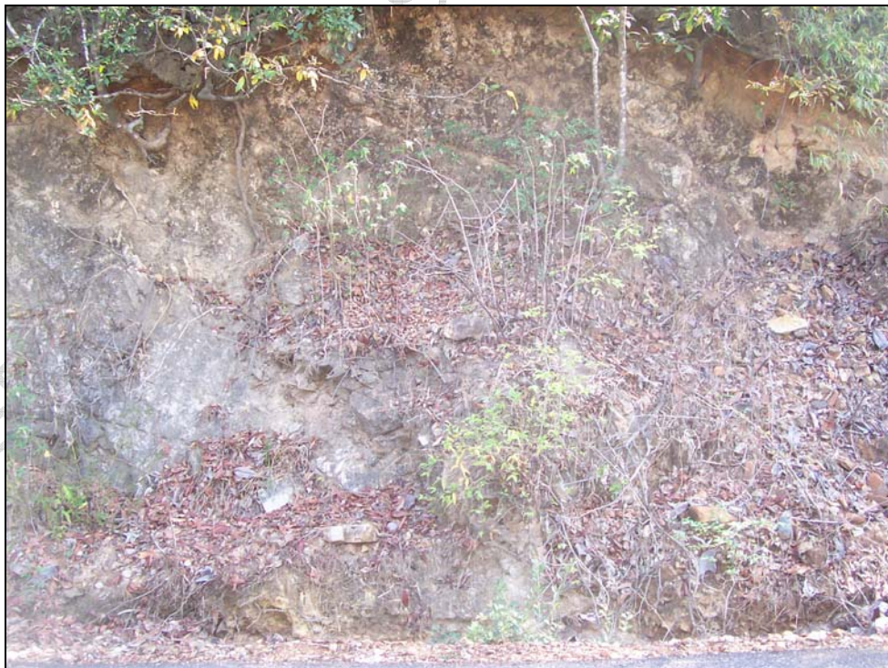
Photo 61: The plan view of rock slide along day lighted plane
