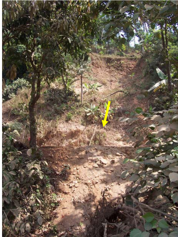
Photo53: Plan view of the reactivated debris slide which has length of 17m
