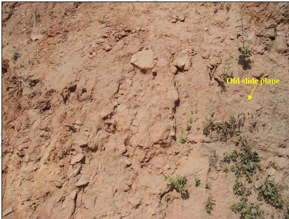
Photo 14: Deeply weathered granite exposed in the slide plane with old slide plane
