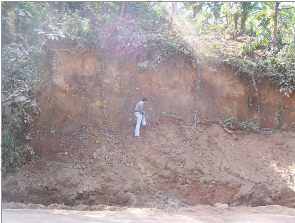
Photo 29: The plan view of the debris slide with crown height of 4m.
