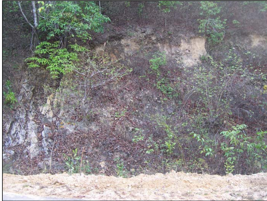
Photo 62: The plan view of the reactivated rock slide along day lighted plane.
