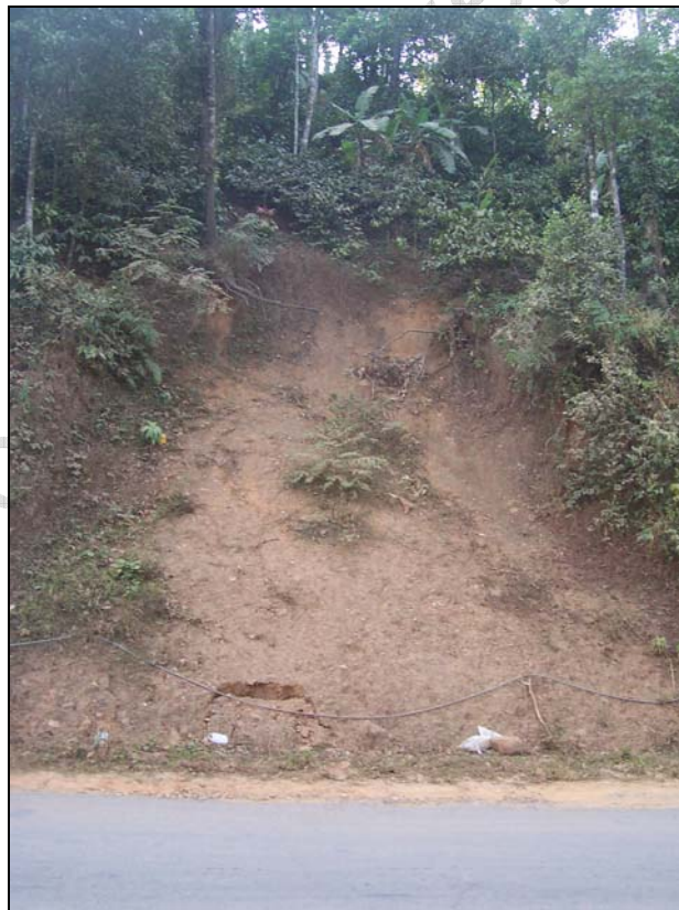
Photo 42: The plan view of the debris slide with huge trees standing on the crown
