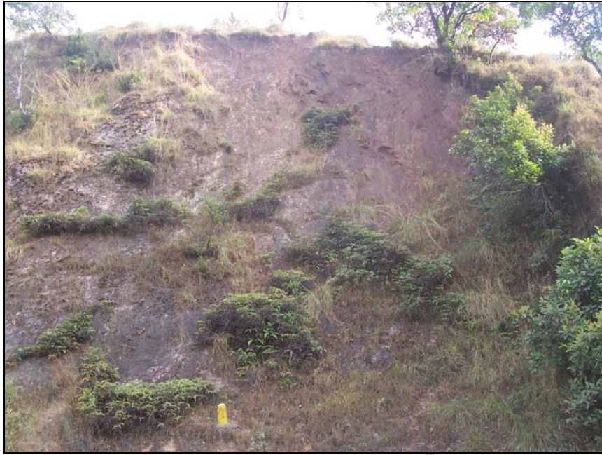
Photo 49: View of the debris slump exposing the bed rock over which it has moved.
