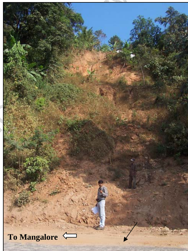
Photo-4: The SH88 was blocked (arrow) and the slided debris was heaped up on the road
