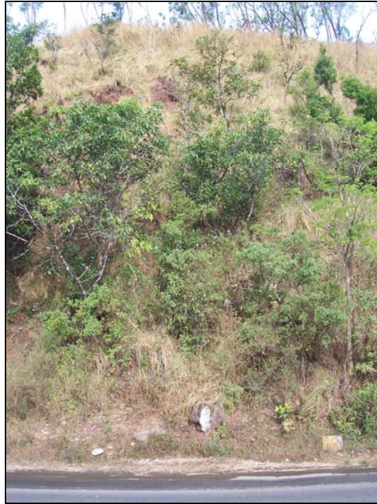
Photo 45: Plan view of the debris slide with exposed weathered granite
