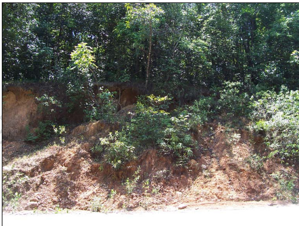
Photo 87: The plan view of the debris slide with accumulation at the toe.
