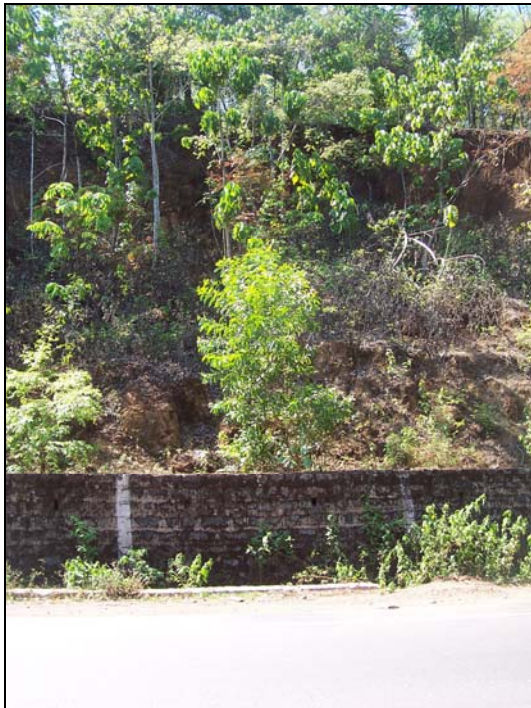
Photo 96: The view of the debris slide with unstable crown
