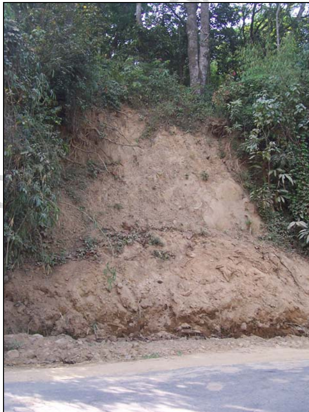
Photo 37: The side view of the debris slide with zone of accumulation
