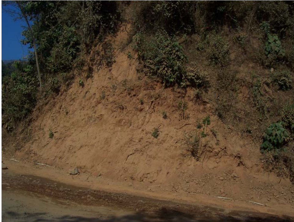
Photo 34: The plan view of the debris slide with unstable crown
