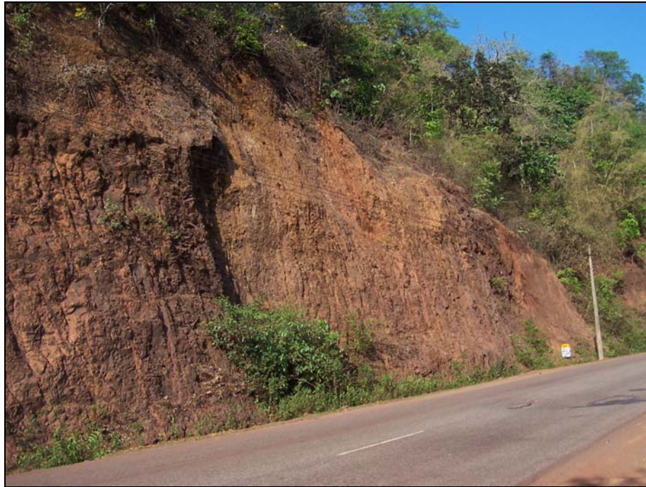
Photo 105: The side view of the reactivated debris slump with steep slope angle
