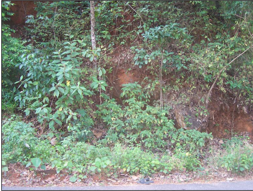
Photo 66: The plan view of the debris slide with exposed bed rock
