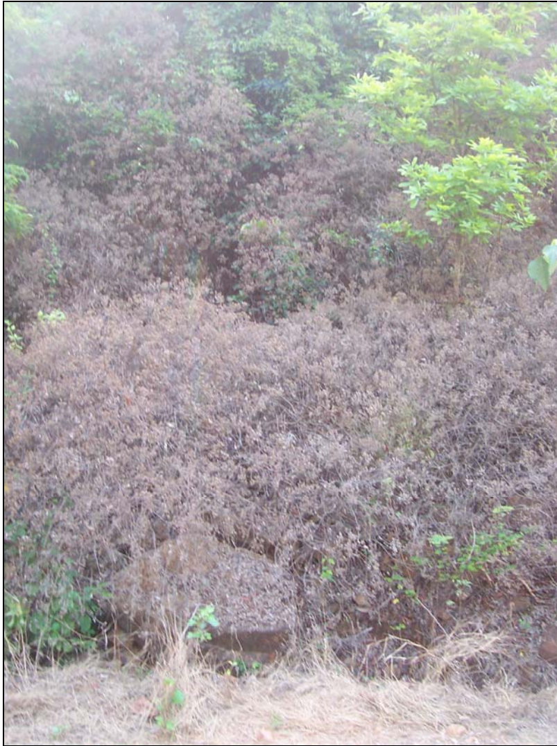
Photo 72: The plan view of the rock slide covered with trees.
